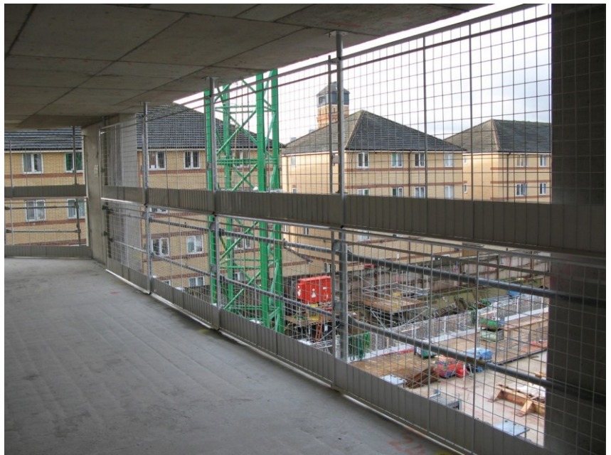
Figure 6: Full height protection with double handrail protection
