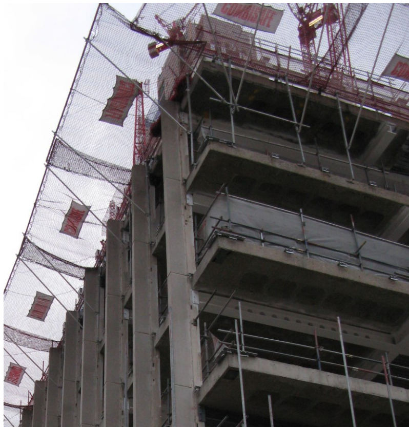
Figure 11: Example of overhead protection fan
