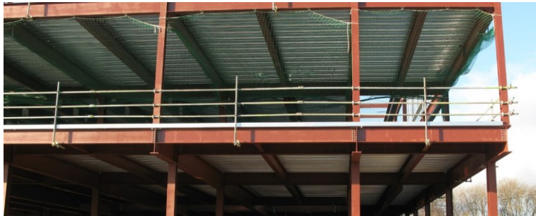
Figure 10: Tube and Fitting Edge Protection
