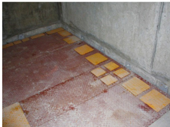
Figure 30: Modular prefabricated deck unit. Reference 3.2.2
