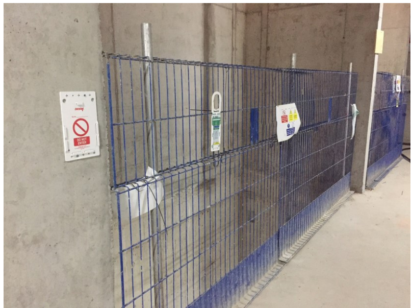
Figure 35: Proprietary Post and Panel at least 1.5 metre high
