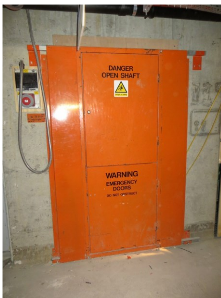
Figure 36: Example of specialist contractor riser protection
