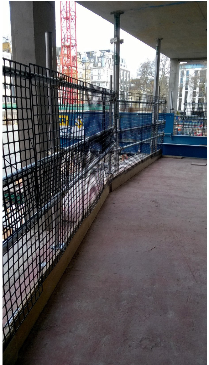
Figure 8: Triple rail tube and fitting edge protection with mesh panel.
