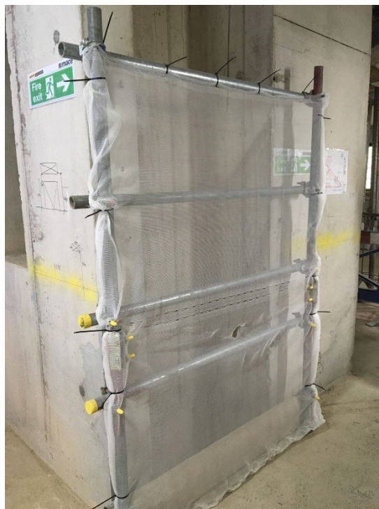
Figure 34: Tube and fitting riser protection
