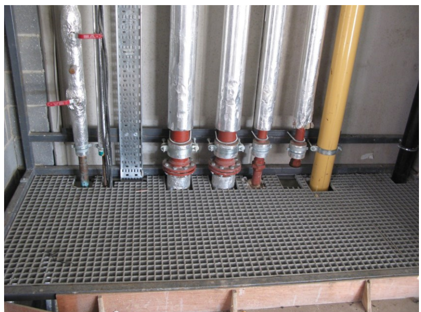
Figure 32: Floor deck installed following frame erection.
