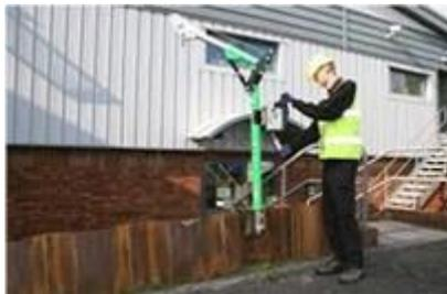
Fig 5 (a) Davit arm for sheet piles
