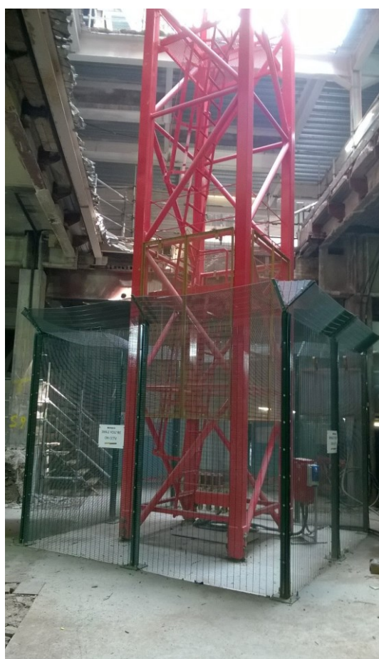
Figure 11: Example of tower crane base setup
