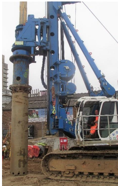
Figure 14: Rotary bored-piling rig showing secondary lifting hook in stowed position on the mast
