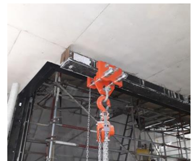
Figure 12: Chain-block attached to lifting beam
