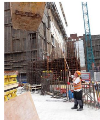
Figure 8: Tower crane carrying load with correct tag line
