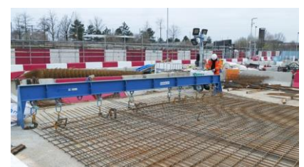
Figure 13: Lifting beam attached to wall re-bar
