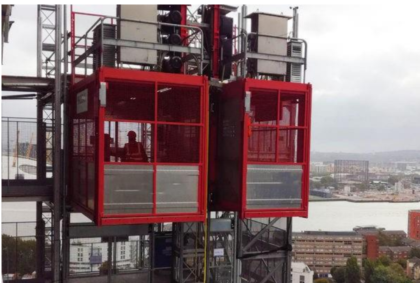
Figure 28: Construction hoist
